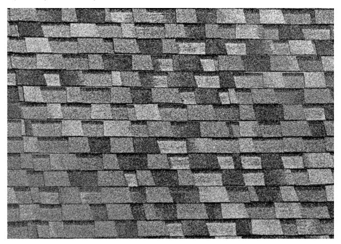
Asphalt shingles are advantageous for a number of reasons. They're inexpensive to manufacture and easy to install making them the most affordable roofing material out there. Asphalt shingle roofs typically last around 15 years which is just longer than the average length of time a homeowners stays in any one home. But for the homeowner looking for more longevity in a roofing product, here are some important things to know.
